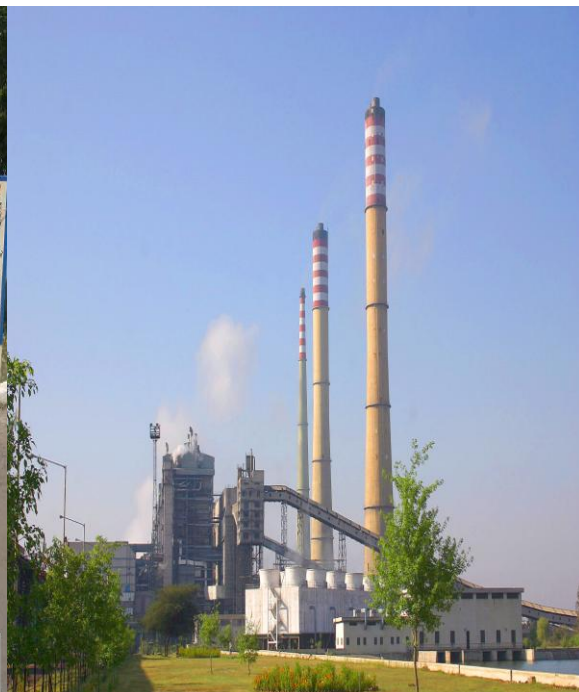
GSECL Thermal Power Station, Panandhro, Kutch
