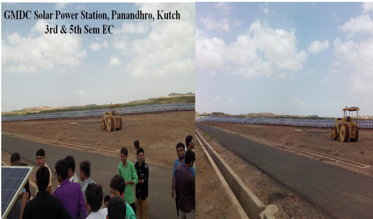
Arrangement of Solar Panel at GMDC Solar Power Station, Panandhro.
